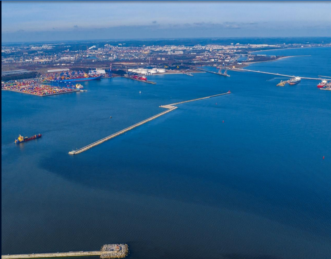
FAIRWAY AND BREAKWATERS Investor: Maritime Office Gdynia
